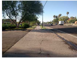
10 SW CORNER LOOKING SOUTH
