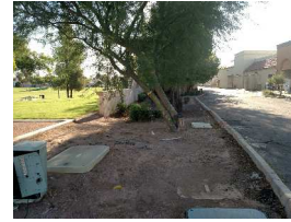
11 SW CORNER LOOKING EAST
