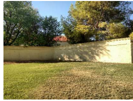
6 SE CORNER LOOKING SOUTH
