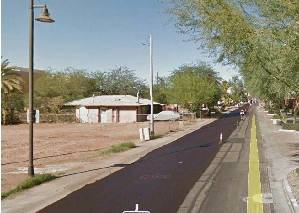
5. SOUTHEAST CORNER LOOKING NORTH
