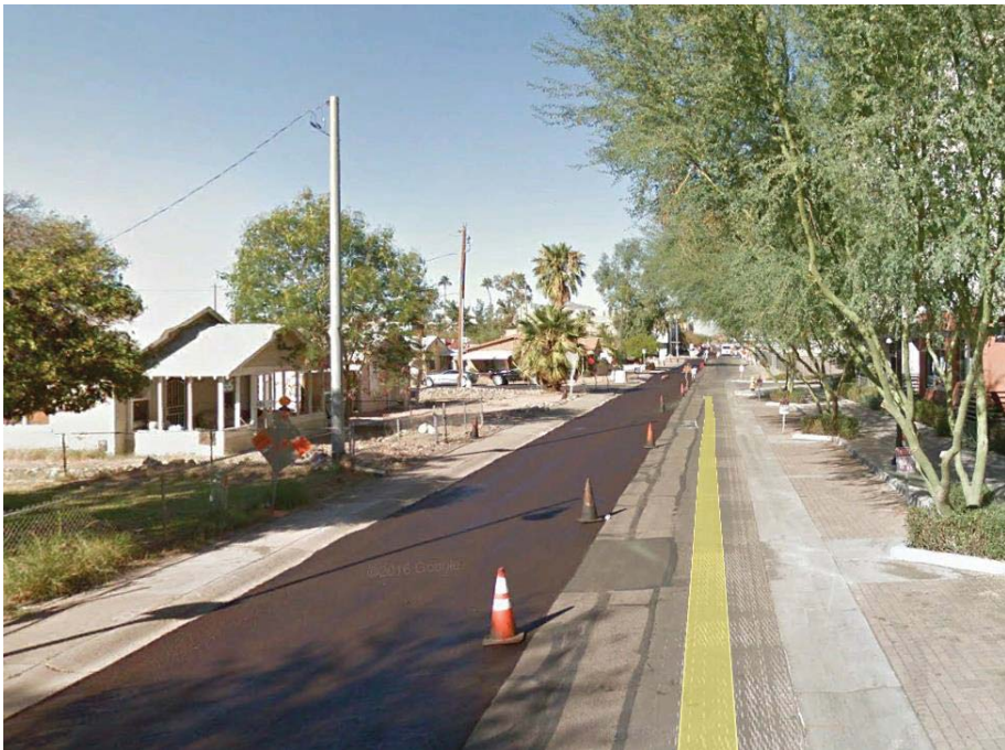
1. NORTHEAST CORNER LOOKING NORTH
