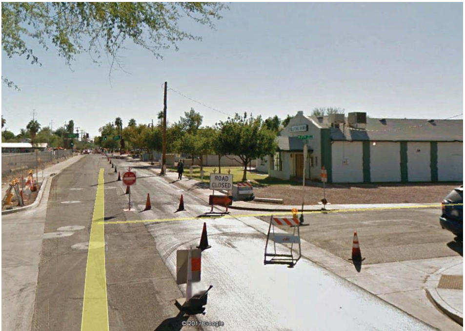
7. SOUTHEAST CORNER LOOKING SOUTH
