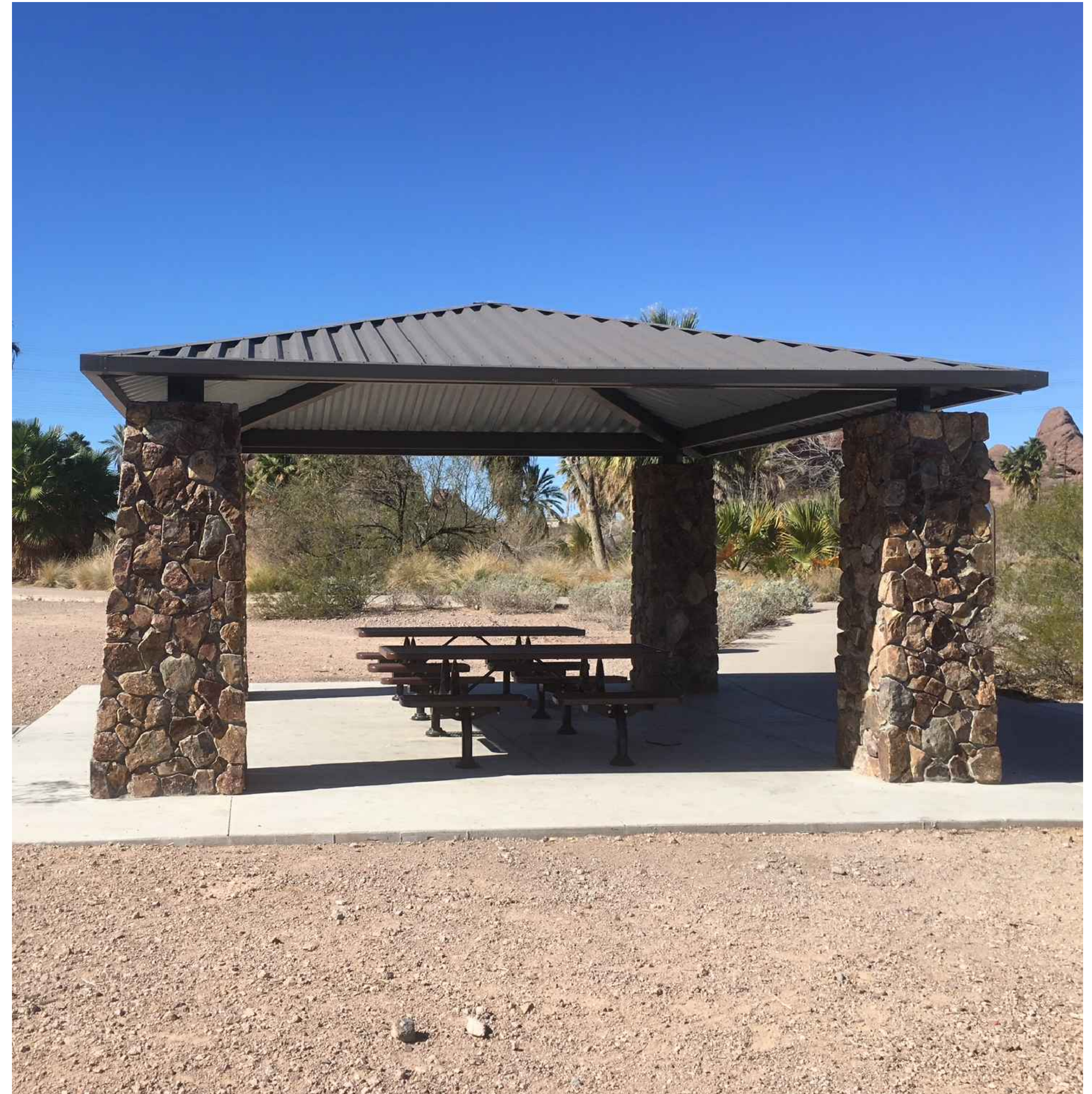
PICNIC RAMADA WITH STONE COLUMNS
