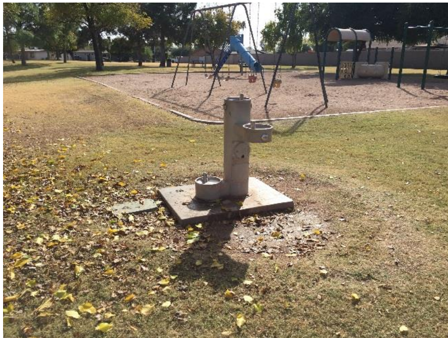
Drinking fountain with no accessible route.
