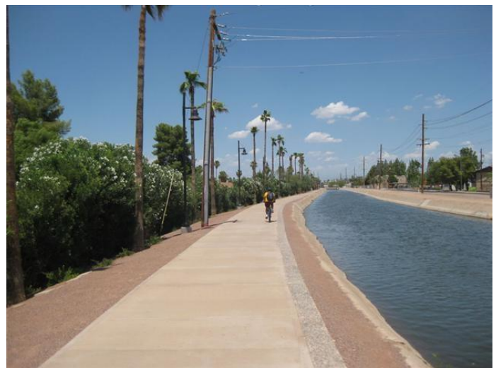
Multi-use Tempe Canal multi-use path
