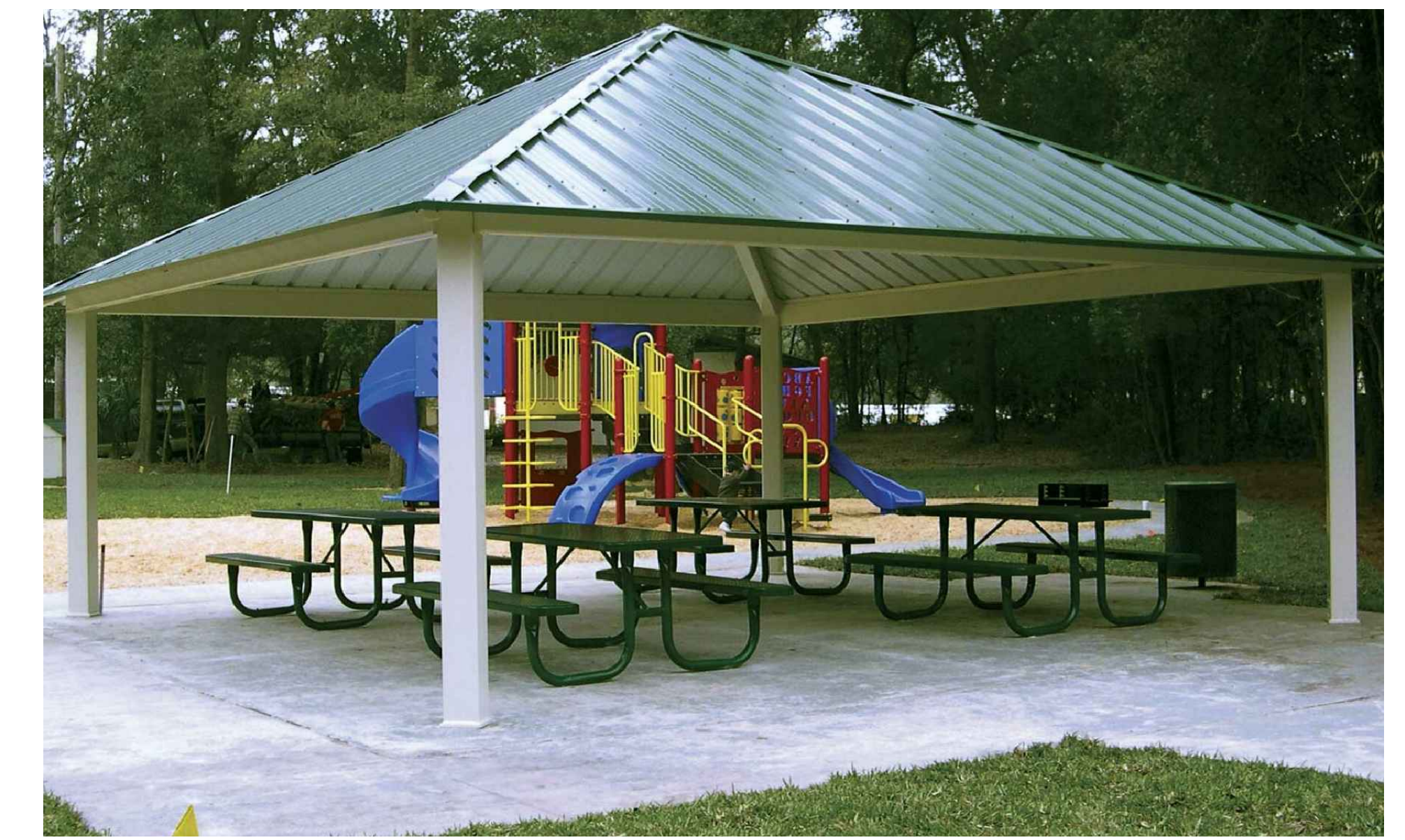
PICNIC RAMADA METAL ROOF STRUCTURE
