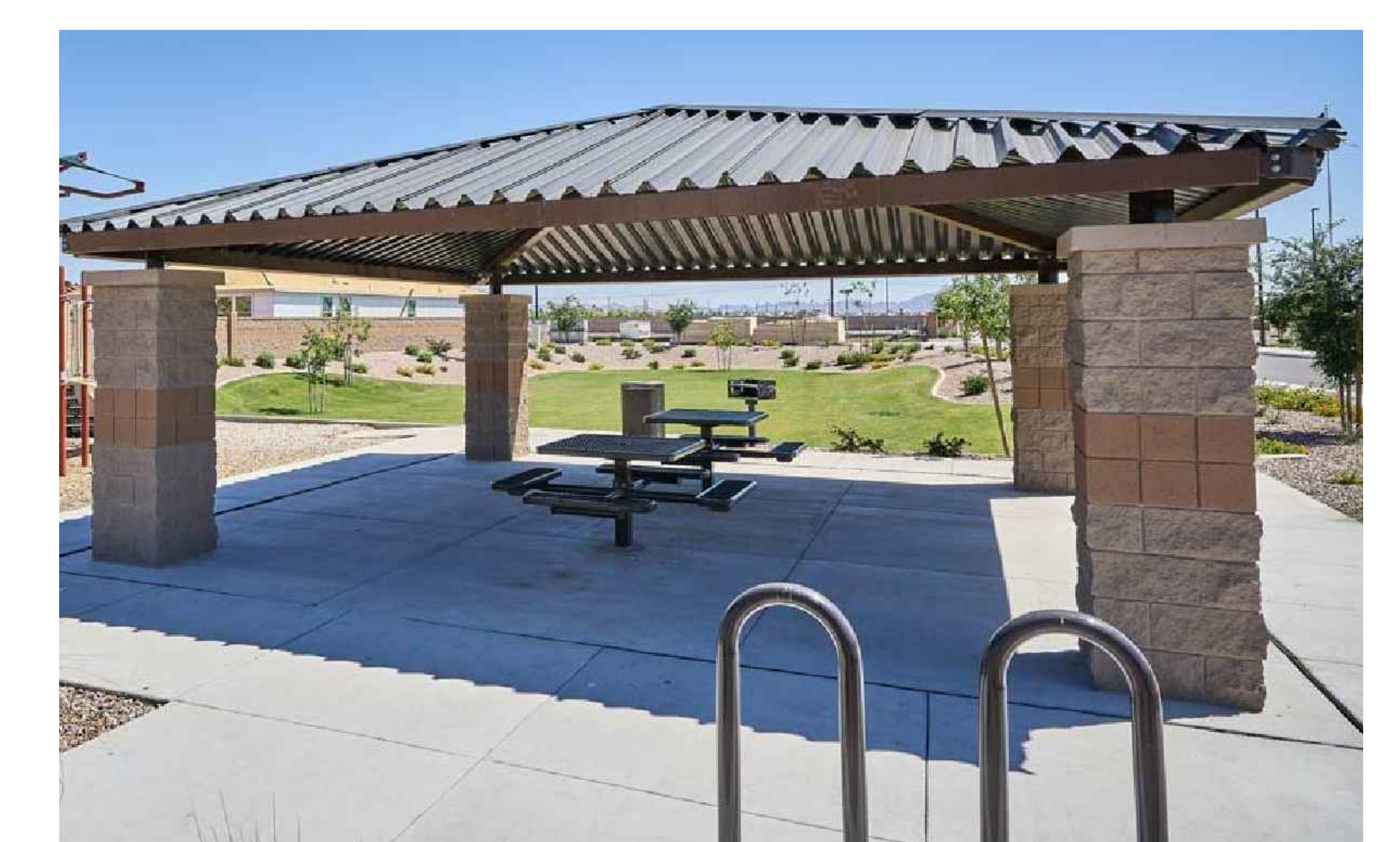
PICNIC RAMADA METAL ROOF STRUCTURE
