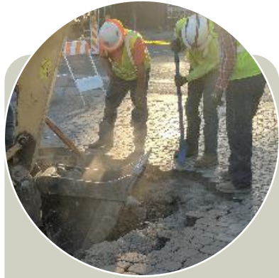
Utility Relocation & CNPA
