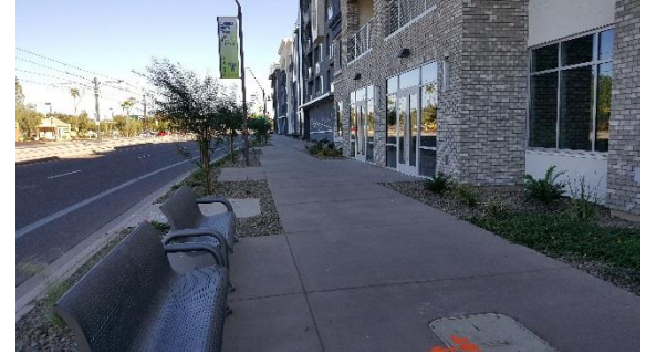
Multi-family development on Apache Blvd . Street level interface
