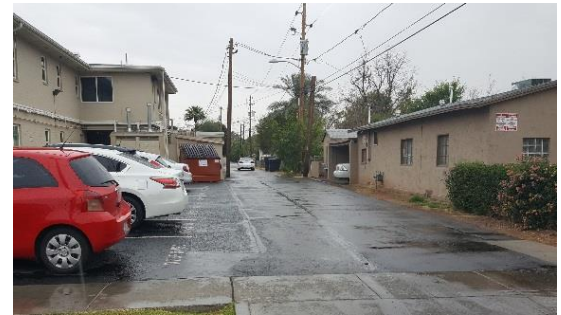
Juxta position of commercial uses with single family development. W. of Mill Ave S. of University Dr.
