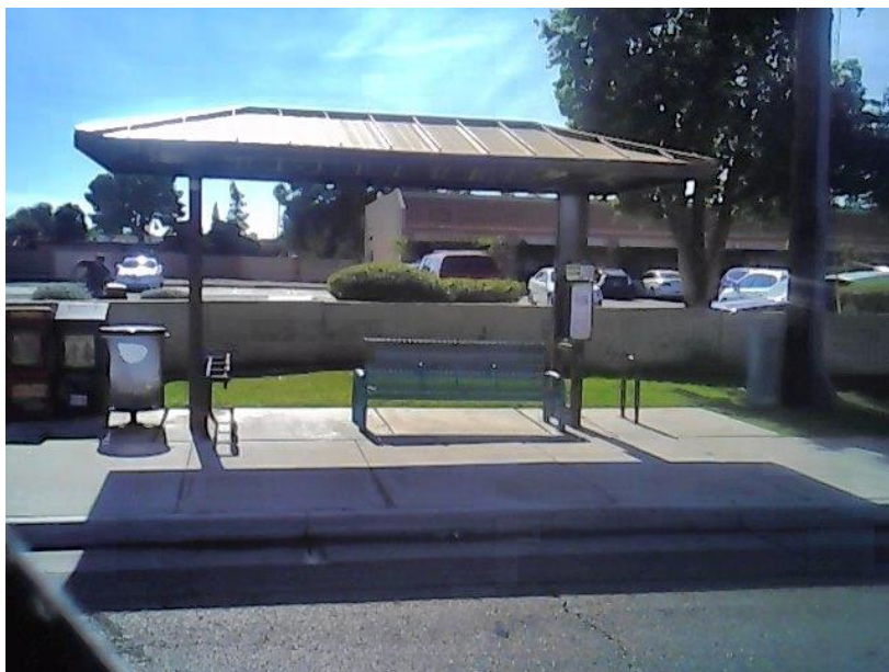
Compliant Transit Stop
