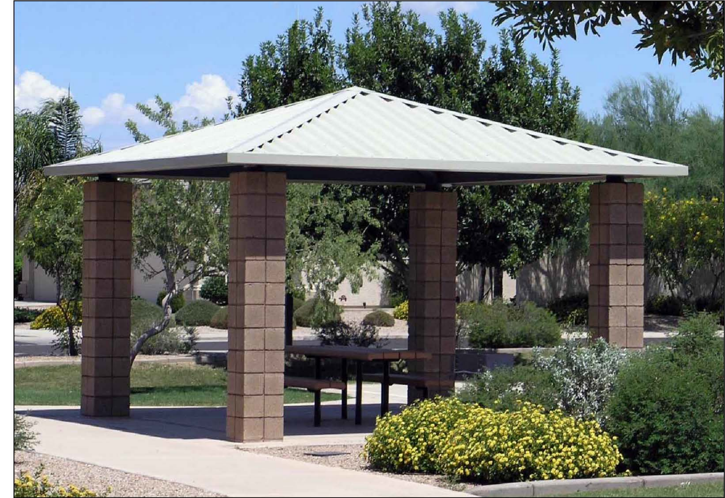
SCoured CMU BLOCK FINISH
