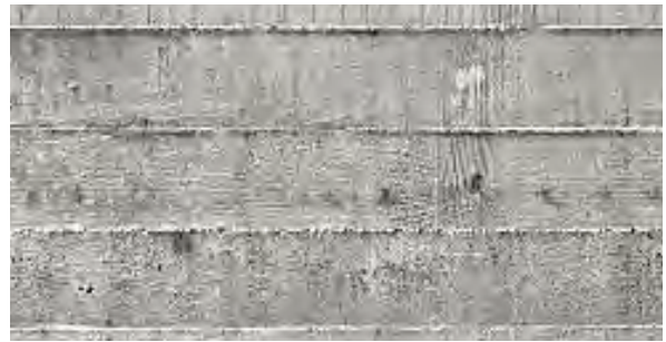
12 CAST IN PLACE BOARD FORMED CONCRETE SITE WALL. COLD GRAY.
