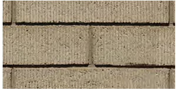
4 8" x 4" x 16" SUPERLITE FOUNDERS FINISH MASONRY BLOCK. COLOR: 'BONE'. RUNNING BOND
