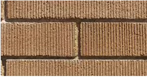
1 8" x 4" x 16" SUPERLITE FOUNDERS FINISH MASONRY BLOCK. COLOR: 'HAYDEN'. RUNNING BOND
