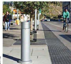
FLUSH PAVING CONDITION
