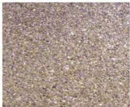
ACID ETCH CONCRETE FINISH
