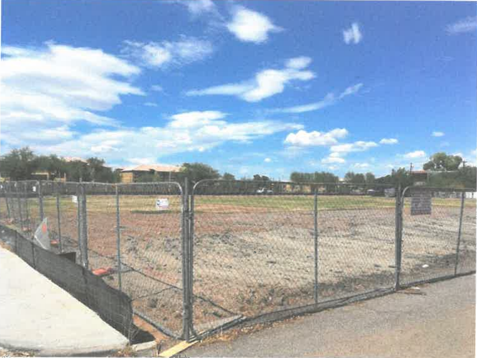
Southwest corner of the site at Gary Drive and the Alley looking northeast
