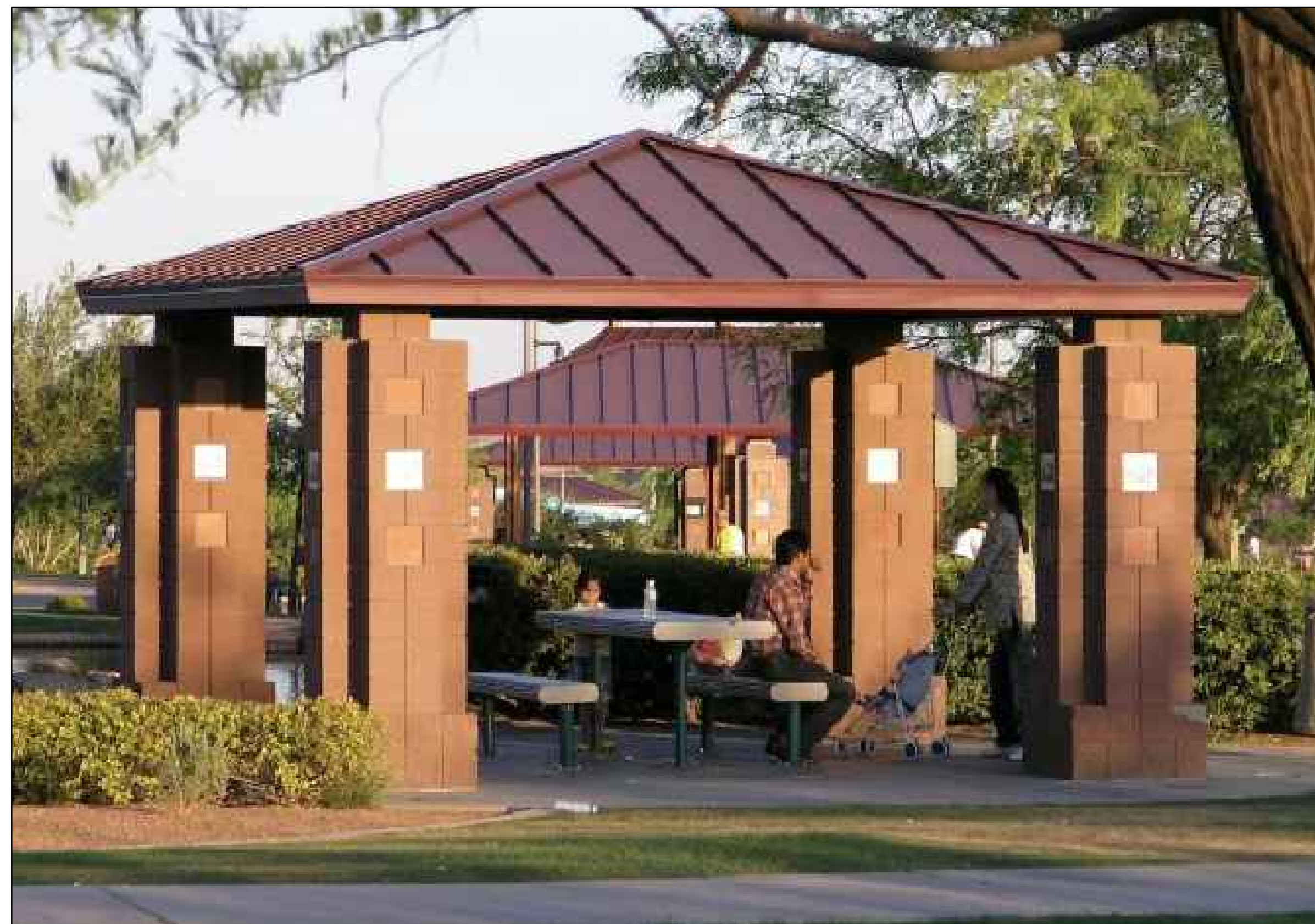
NOTCHED CMU BLOCK FINISH
