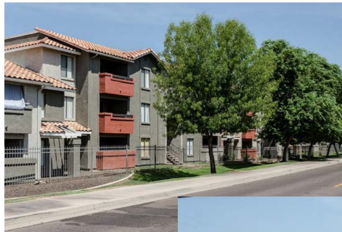
Sonterra Apt.'s on the West
