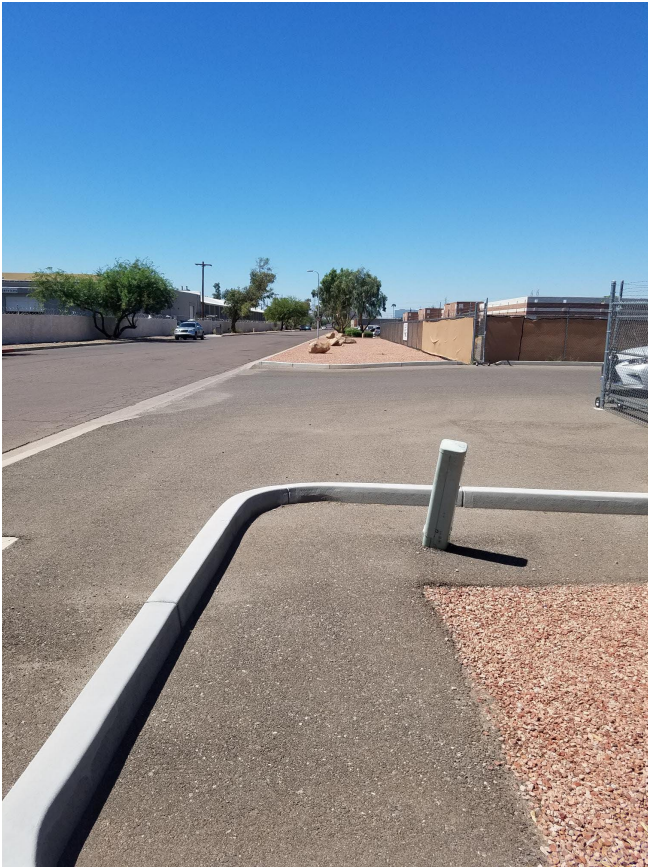
PICTURE 3 SE CORNER LOOKING WEST
