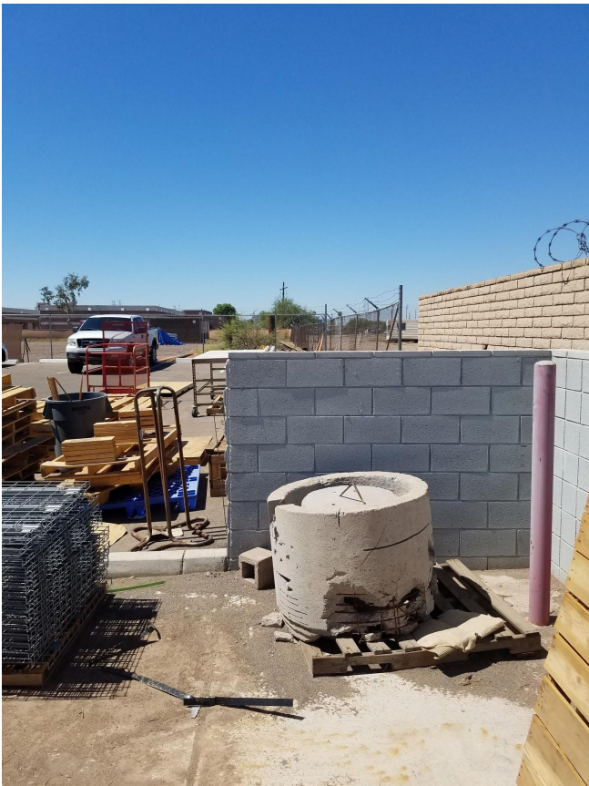
PICTURE 2 NE CORNER LOOKING WEST
