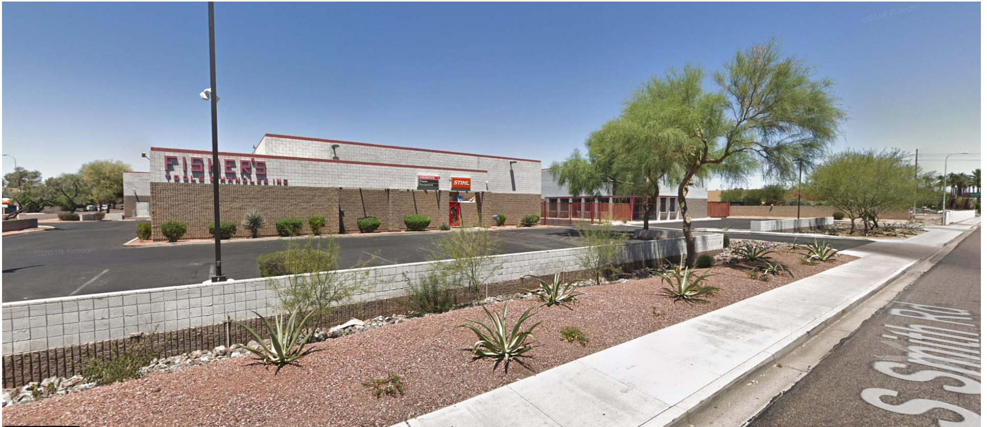
PICTURE 9 VIEW OF EXISTING FISHER'S TOOLS PHASES FROM SMITH ROAD
