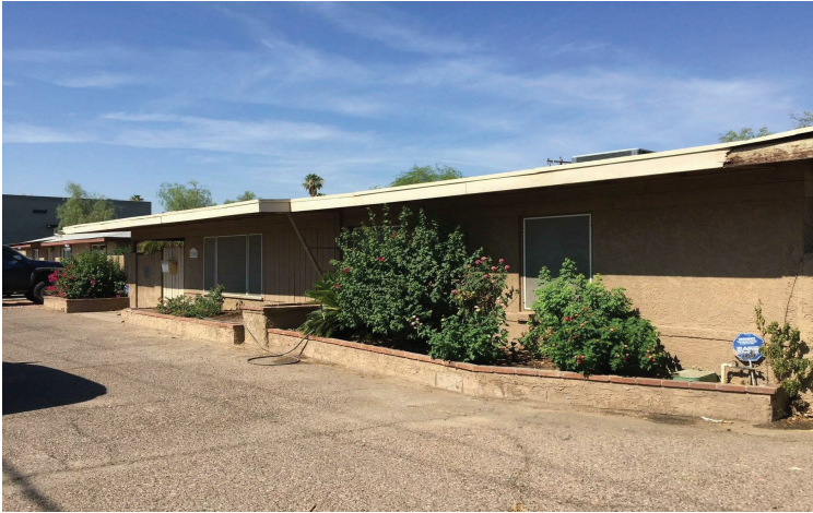
FRONT ELEVATION LOOKING SOUTHWEST
