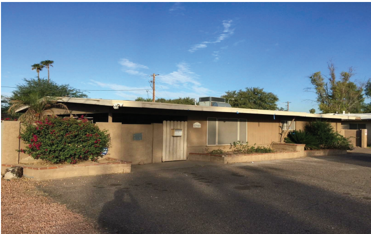
FRONT ELEVATION LOOKING NORTHWEST
