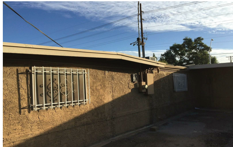
REAR YARD LOOKING TOWARD EAST
