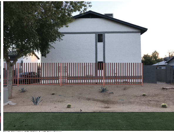
North Elevation of Building-A with New Fence
