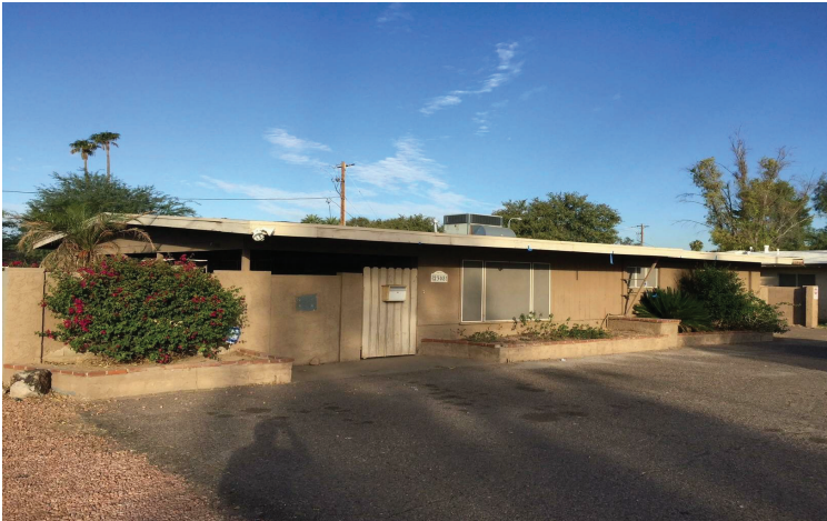
FRONT ELEVATION LOOKING NORTHWEST
