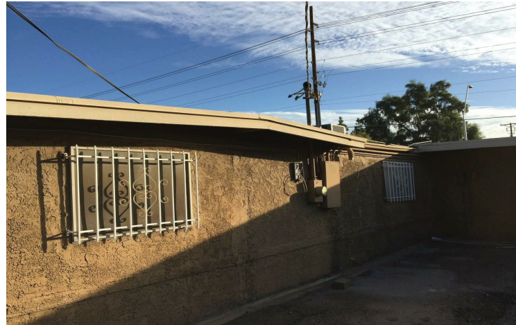
REAR YARD LOOKING TOWARD EAST
