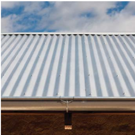
5 GALVANIZED 24 GA CORRUGATED STEEL DECK ROOFING
