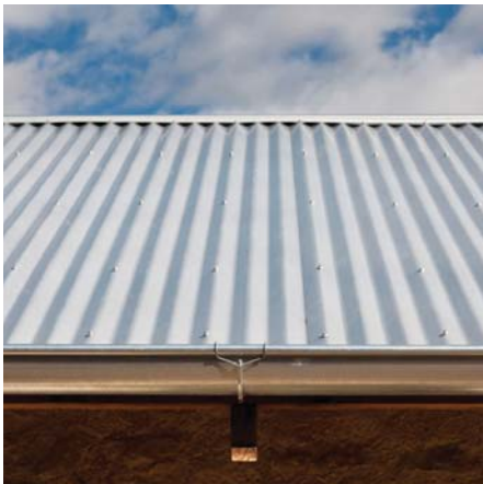
5 GALVANIZED 24 GA CORRUGATED STEEL DECK ROOFING
