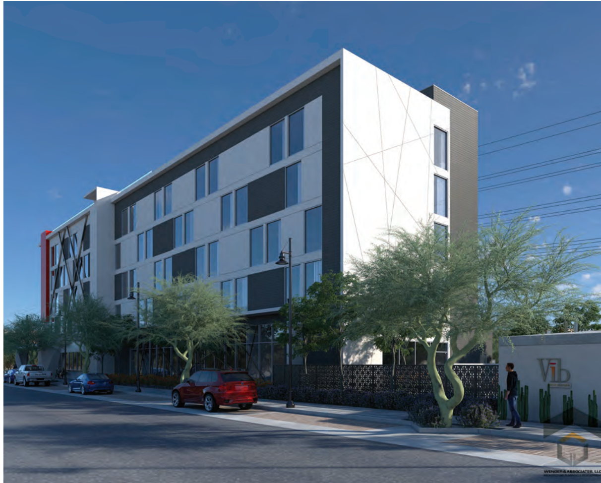
VIEW OF WEST AND SOUTH ELEVATIONS
