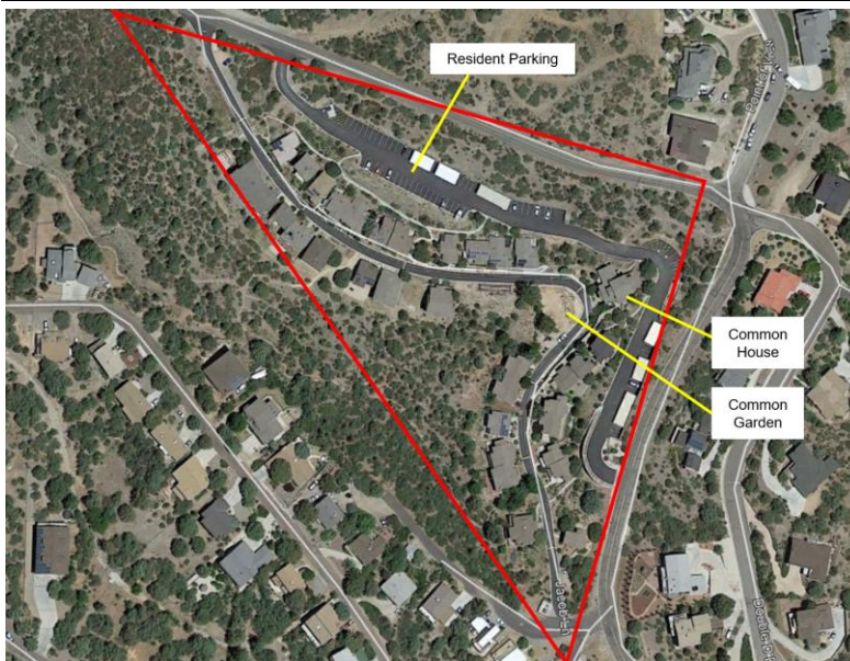
Figure 18: Aerial View of Manzanita Village
