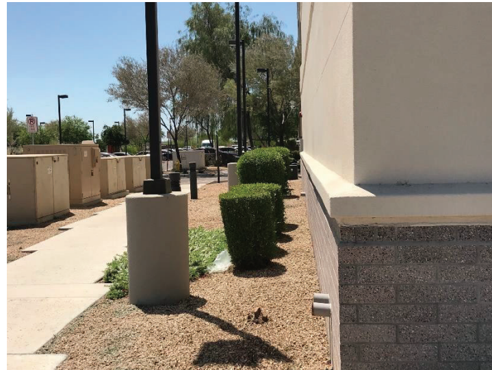
19 | Southeast corner looking South
