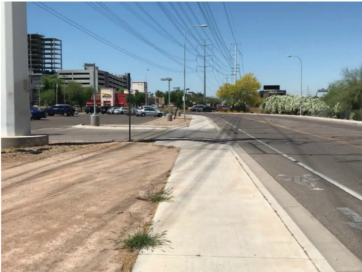
4 | Northwest corner looking West
