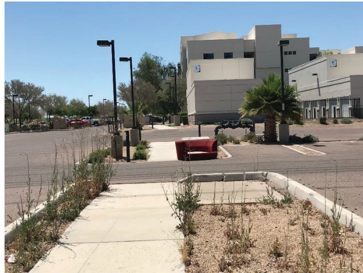
13 | Northeast corner looking South
