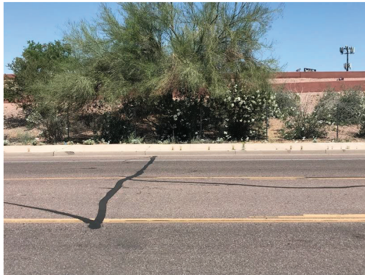
5 | Northwest corner looking North
