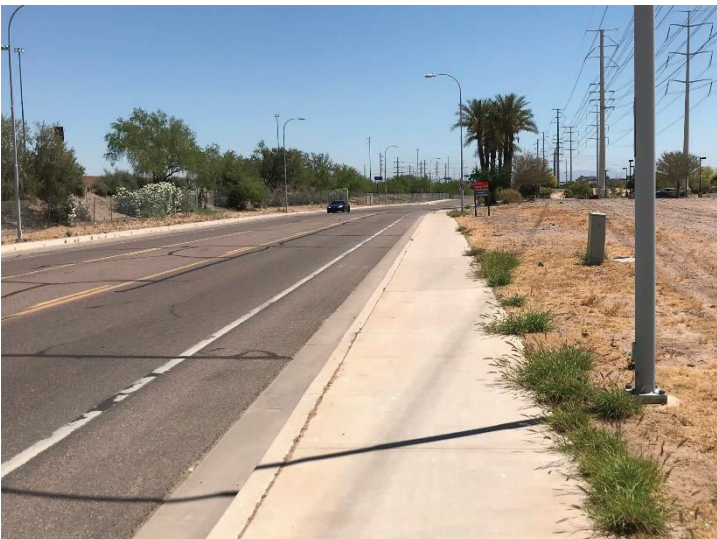
6 | Northwest corner looking East
