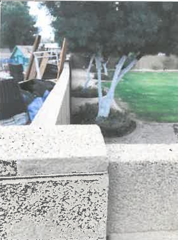
June 20, 2018: Block fence bowing due to granite slabs and debris leaning on fence.
