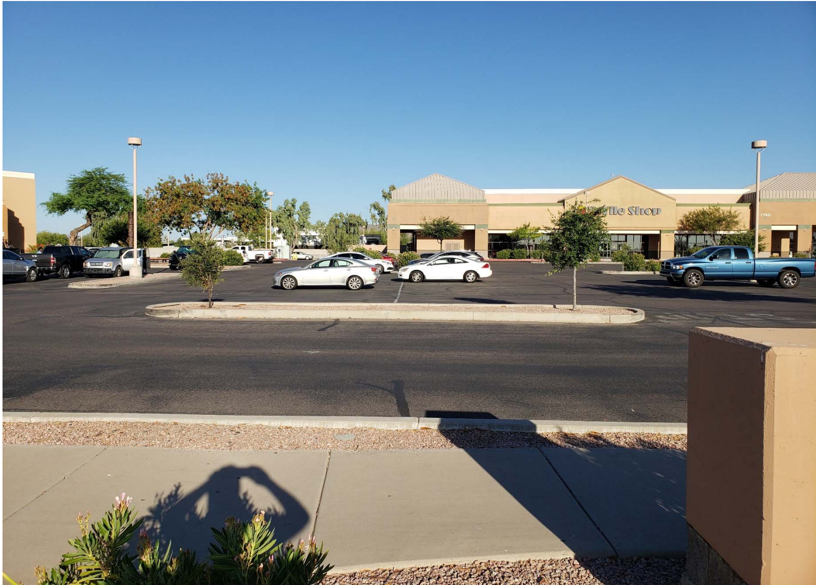
PICTURE #12 – VIEW TO THE WEST FROM THE NORTHWEST PROPERTY CORNER
