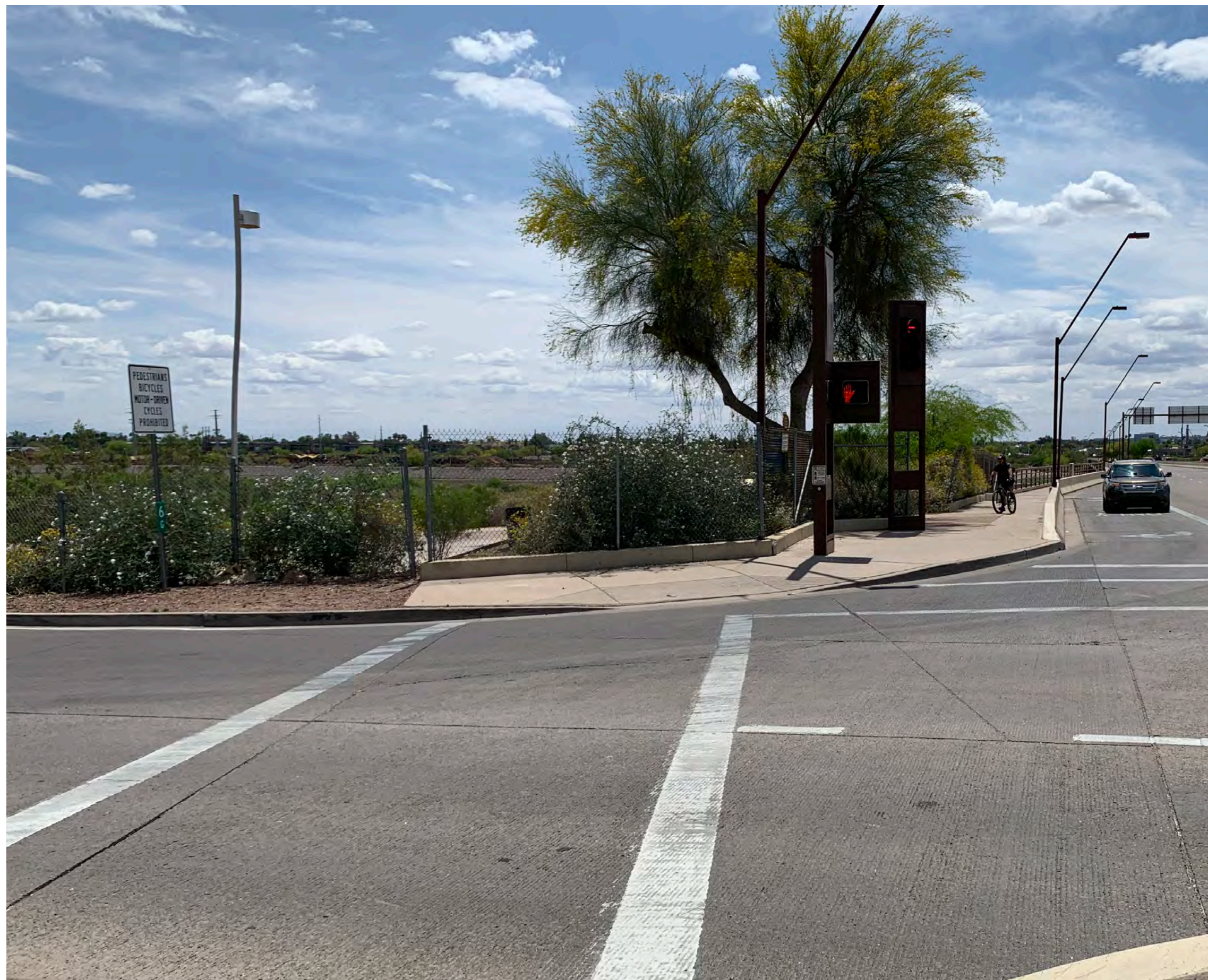
N. PRIEST DR AND SR 202L EB ON-RAMP - EXISTING PED CROSSING
