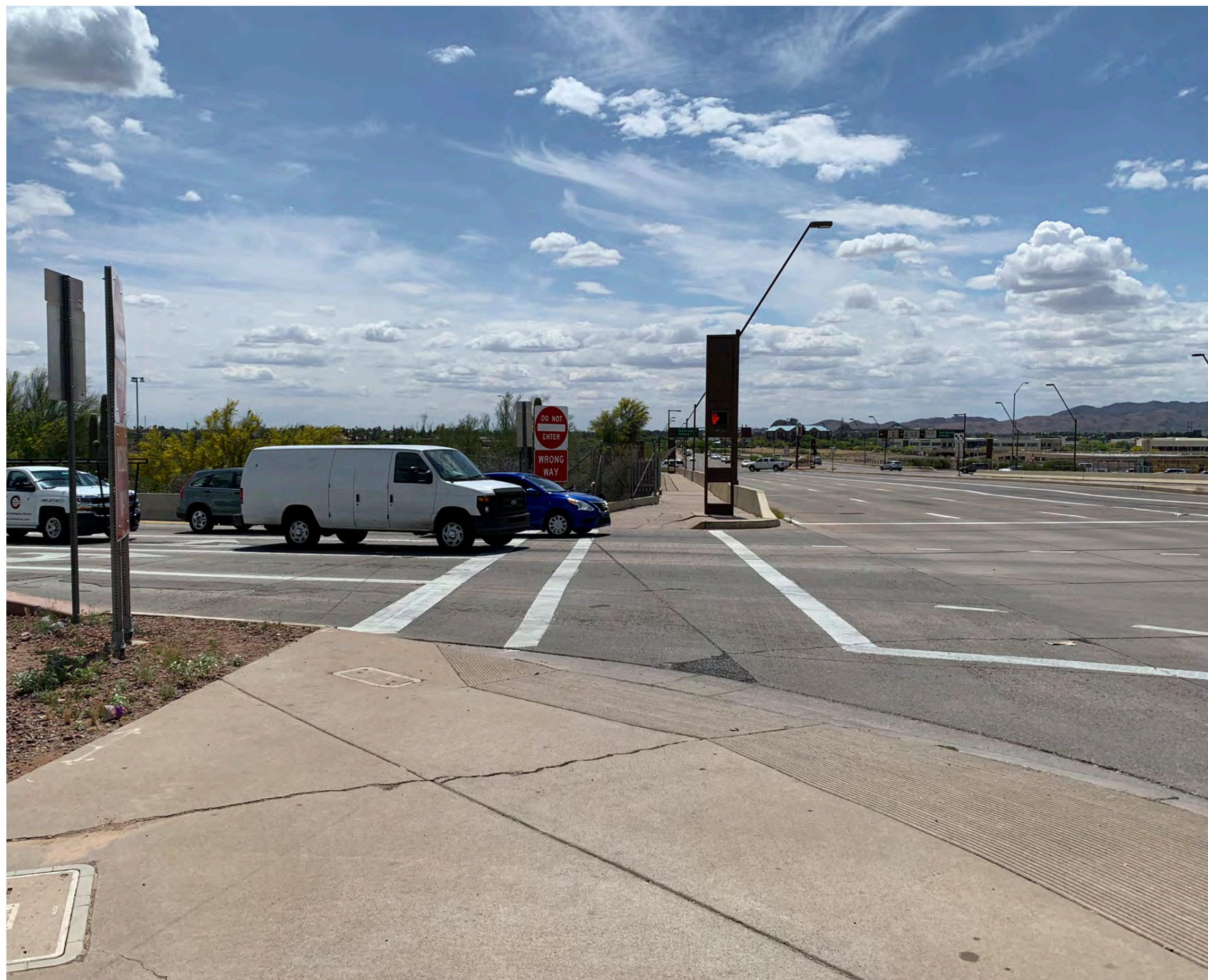
N. PRIEST DR AND SR 202L WB OFF-RAMP - EXISTING PED CROSSING
