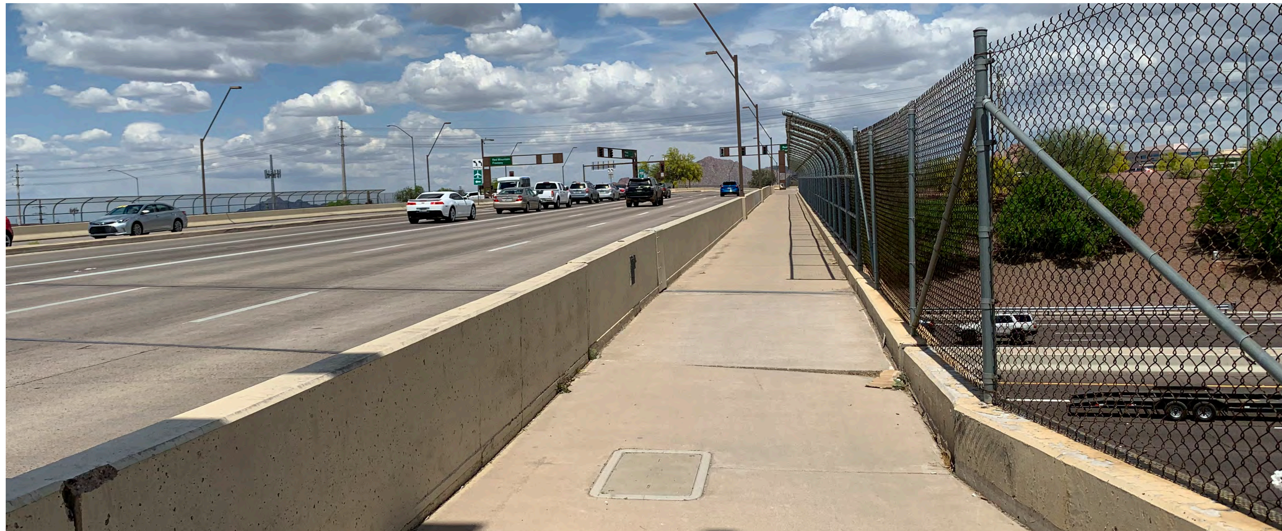
N. PRIEST DR - EXISTING SIDEWALK LOOKING NORTH
