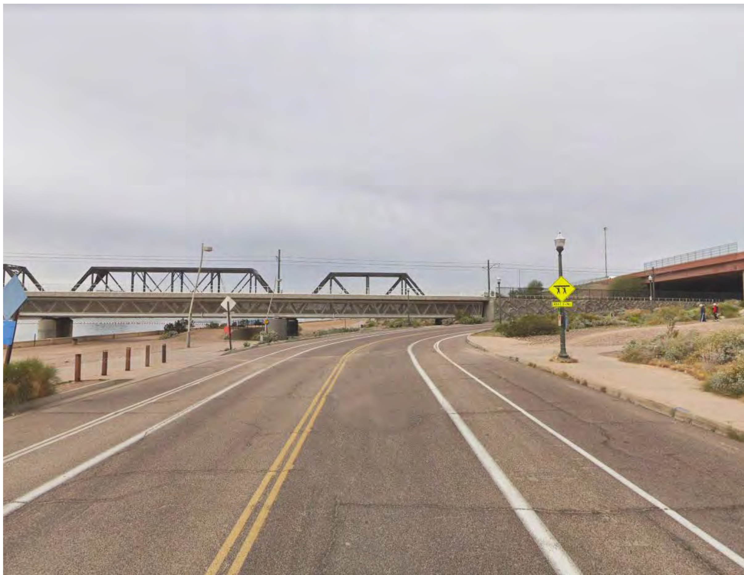
LAKE VIEW DR - EXISTING PED CROSSING
