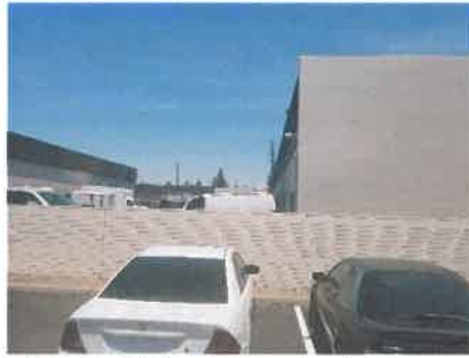
Photo 9: NE corner looking North
