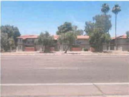
Photo 4: NW drive looking West
