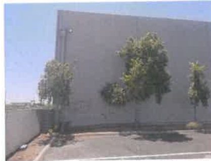
Photo 15: SE corner looking South
