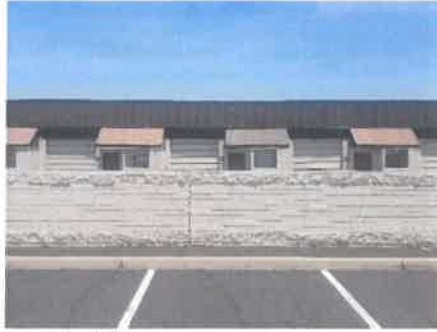
Photo 5: Middle north looking North
