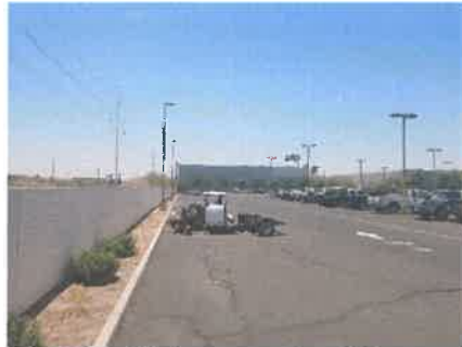
Photo 11: NE corner looking South
