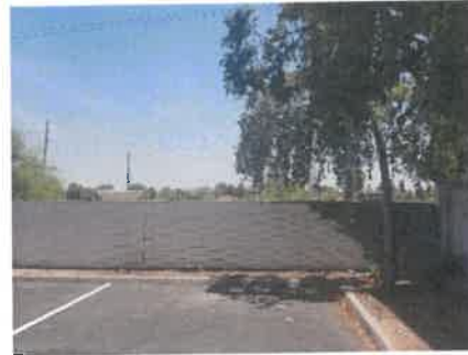
Photo 14: SE corner looking East
