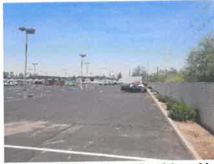
Photo 13: SE corner looking North
