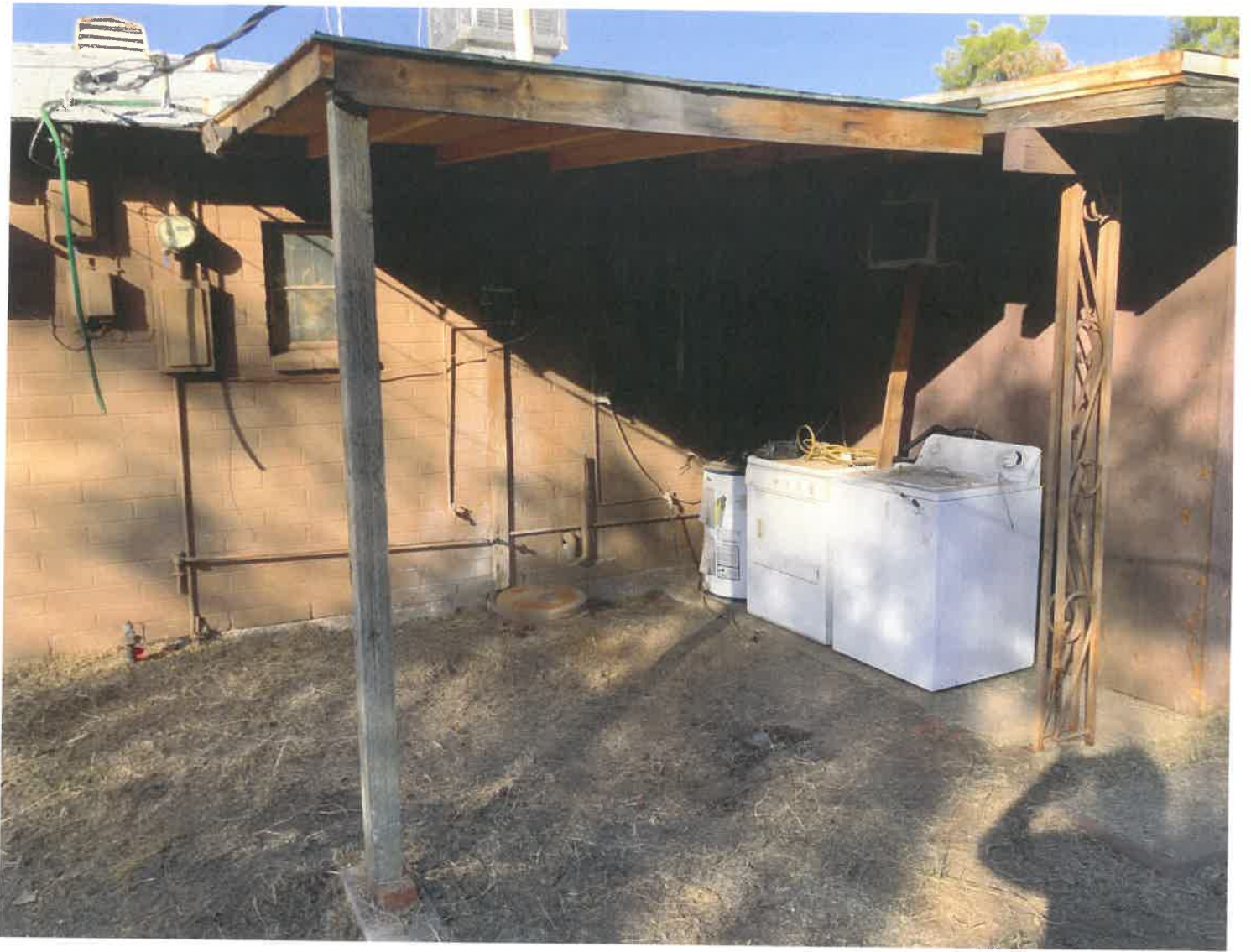
5, WASHER, DRYER, HOT WATER TANK
