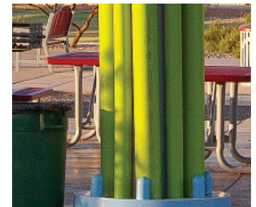
Painted Steel Pipes
