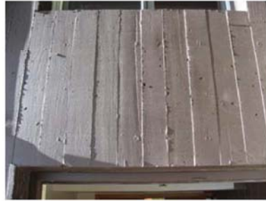
Board Formed Concrete
