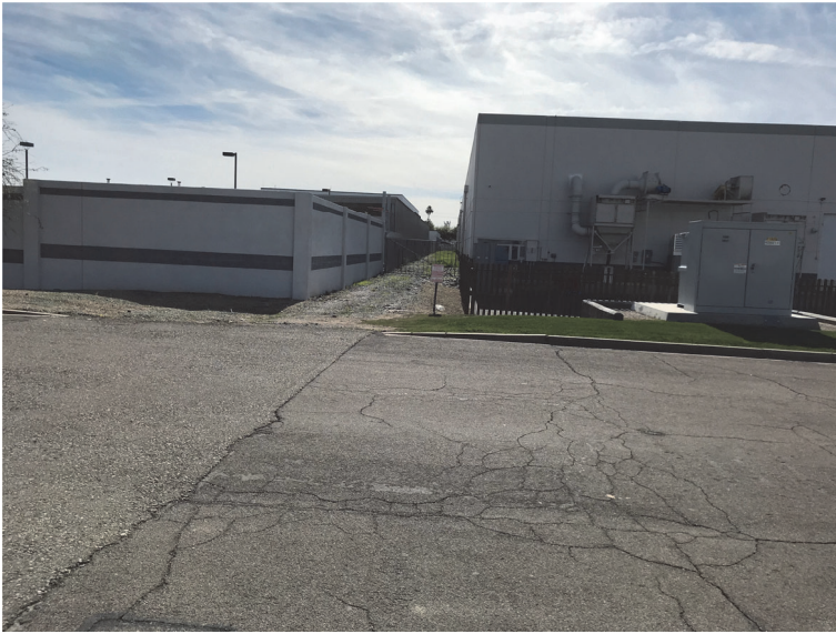
A. FACING SOUTH
