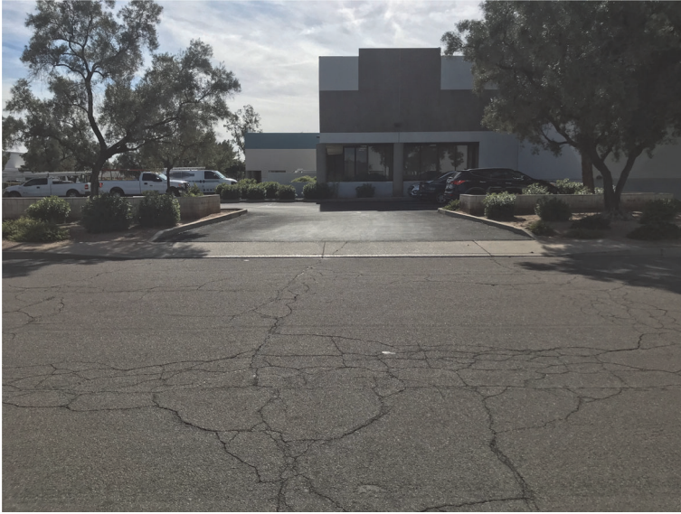
A. FACING SOUTH
