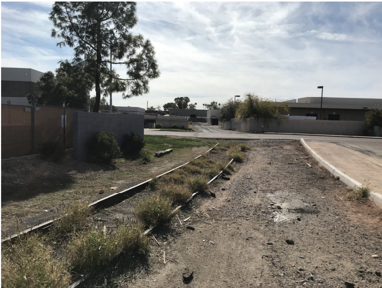
C. FACING SOUTH
