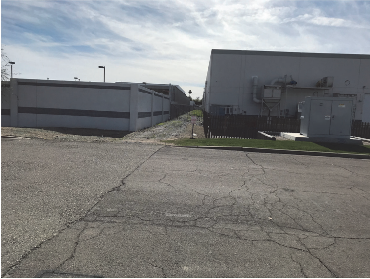
A. FACING SOUTH
