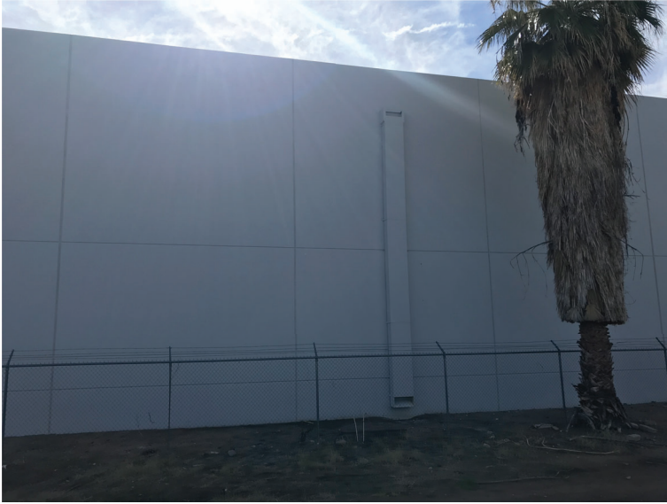
A. FACING SOUTH
