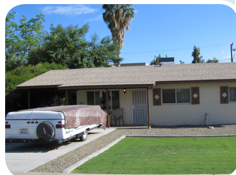
Asphalt shingles are a prominent feature of historic homes in the neighborhood. These must be maintained in order to have a contributing property.
