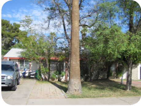
Porch screens that do not allow visibility of the doors and windows is not in compliance with the HPC standards of a historic contributing property.
