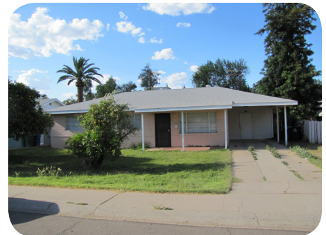
This entry porch maintains the original features of the Ranch Home. The 4x4 support column is a distinct feature unique to this house type.
