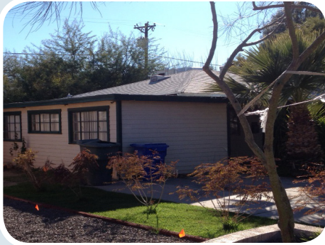
This is an example of a carport enclosure that was done during the period of significance and is now historic in its own right.
