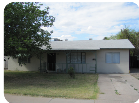
When enclosing a carport, it is important that the new construction does not encroach into the historic setbacks. This is an example of sensitive construction respecting the original plan.
