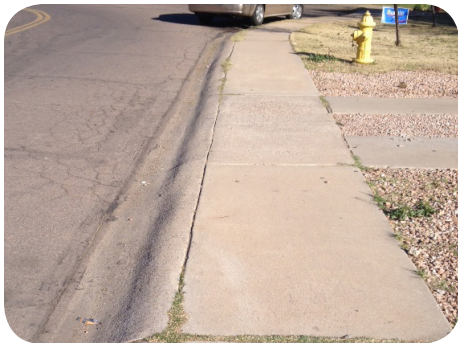
Typical 4' sidewalk and rolled curb/gutter in Tomlinson Estates.
