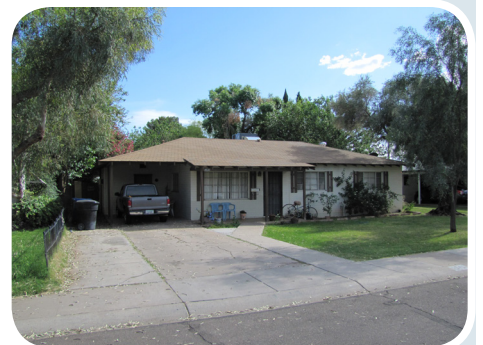
This entry porch is an example of the type of porch built for the Early Transitional Ranch style home.
