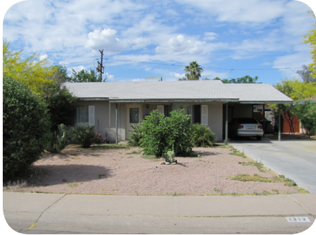
The carport on this property is set back behind the main line of the house in order to not breach the historic setback.
