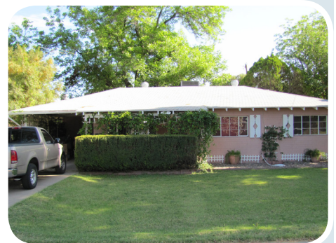
One type of shutter pattern utilizes the two vertical wood slats connected by two horizontal pieces.
