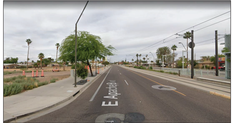
Location A, View 2 looking east
