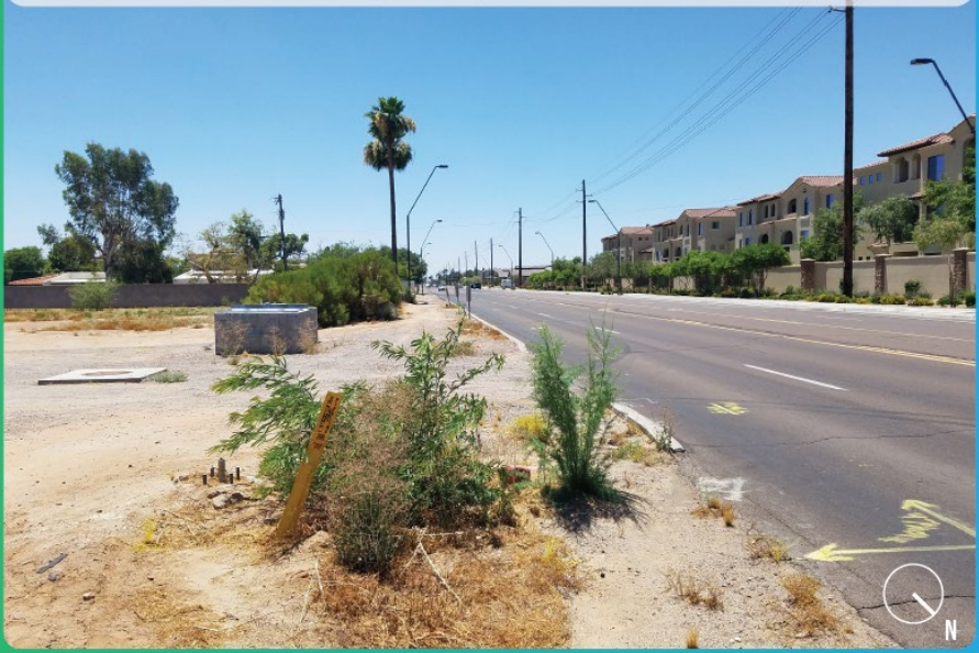
LOOKING SOUTH. MISSING CURB, GUTTER, SIDEWALK, BIKE LANES ALONG PRIEST DRIVE SOUTH OF WARNER
