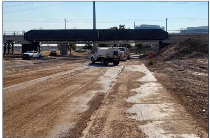
Current Condition of Rio Salado Parkway (Looking East Towards UPRR Bridge)
