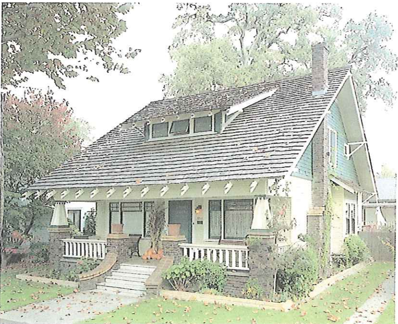
Bungalow in Sacramento, California. With a fringe of rafter tails overhanging its porch and dormer, this house looks as if it had stepped out of the pages of a how-to-plan book. Creating a variety of textures, both brick and buff-colored siding complement the shingled and wood siding. An English carpenter named Jennings created the house and left behind a detailed journal of building expense as a documentary record for the first owners. A large oak tree has grown from the spot that Mr. Jennings and his English bride planted the year their son was born. The son still lives up the street, and has provided the current owners with much house and family lore.
