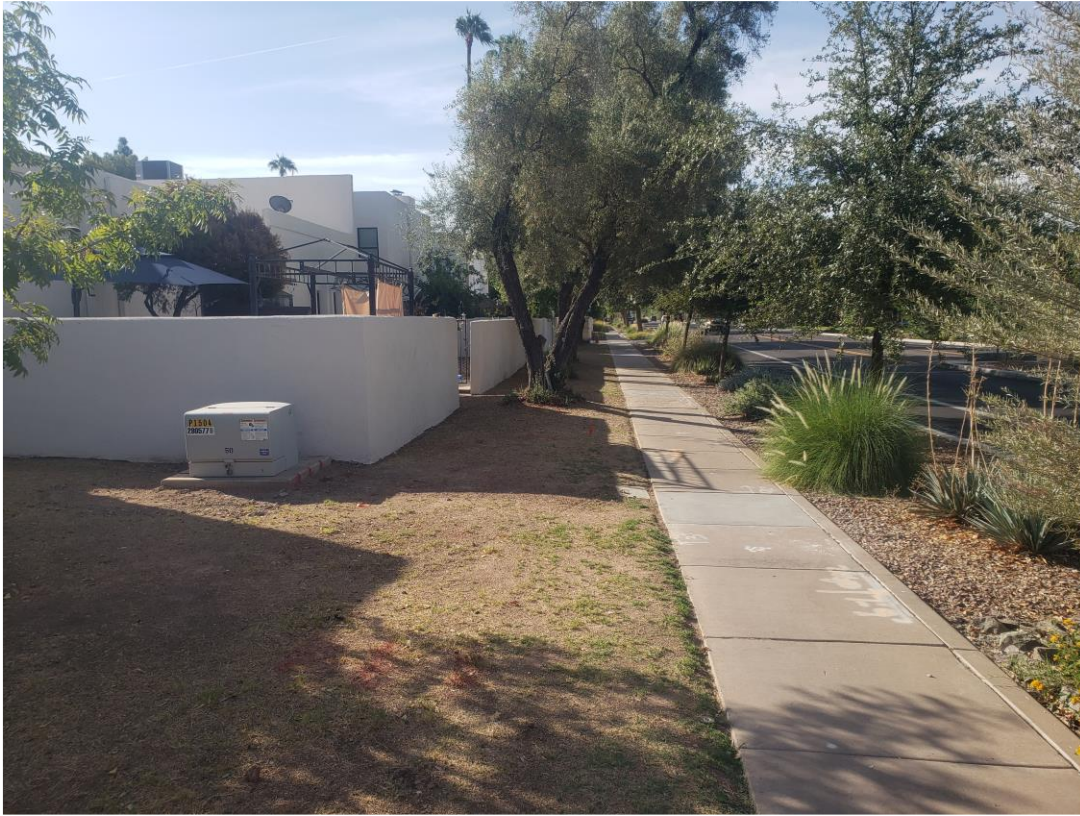
Picture 1 of 4: From the northwest corner of the property, facing south. The near side of the patio wall will be altered so that, after going behind the SRP transformer, it extends further north.
