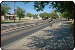
Ramped Bike Lanes
