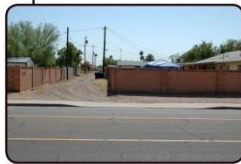
Curb Cut & Alley Not Aligned
