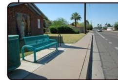
Uncovered Bus Stop
