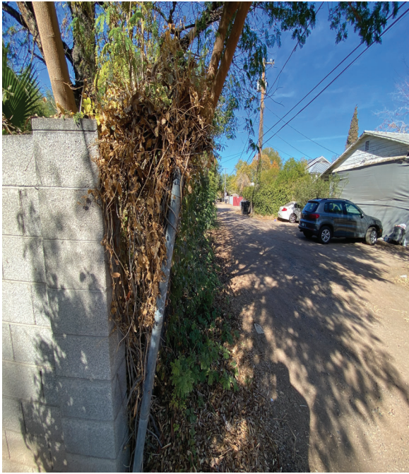
NE Corner - Looking North NE#1N
