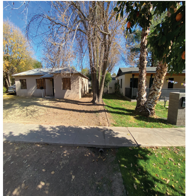
SW Corner - Looking East SW#2E
