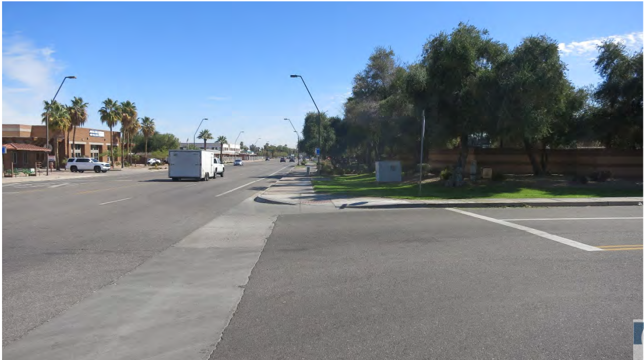
6. Northeast corner looking East.
