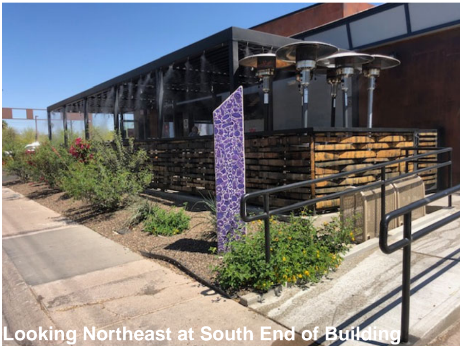
Looking Southeast at South End of Building
