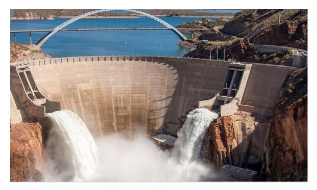
Although the height of the dam was increased by 77 feet, NCS storage exists only in the first 15 feet of the new dam. Above NCS is Flood Control Space (FCS) and the Safety of Dams Space. Due to the constraints of the current operation manual for the dam, water is not routinely stored in either FCS or Safety of Dams space behind the dam.
