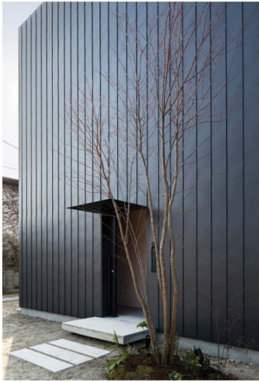
MTL-1: FLUSH FLAT SEAM INTERLOCK SYSTEM COLOR: CHARCOAL GRAY
