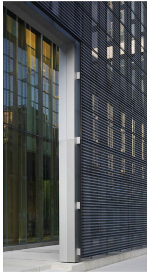
MTL-2: PERFORATED BOX RIB METAL PANEL COLOR: CHARCOAL GRAY
