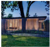
FENCE-1: BLACK 1 1/2" DIA PIPE FENCE @ 5" OC
