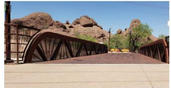
Figure XX Pedestrian bridge over the canal: compatible color, material durability, and massing
