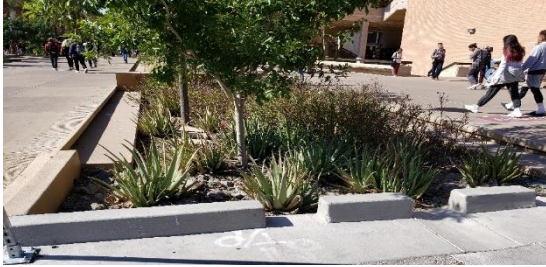
Rainwater redirect to landscaping
