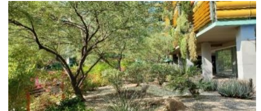
Green roof, and walls
