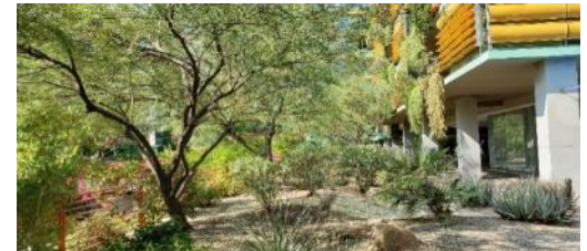
Green roof, and walls
