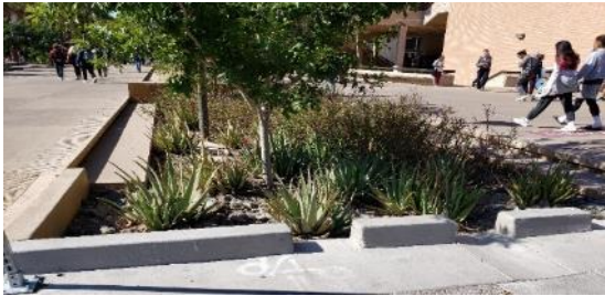
Rainwater redirect to landscaping
