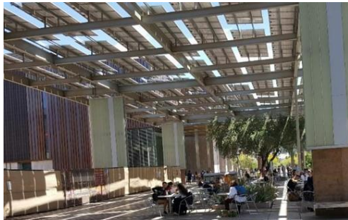
Shading of walkways by solar panels
