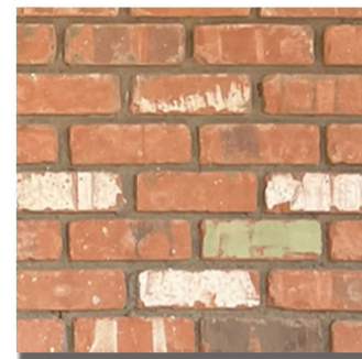
EXISTING BRICK VENEER
