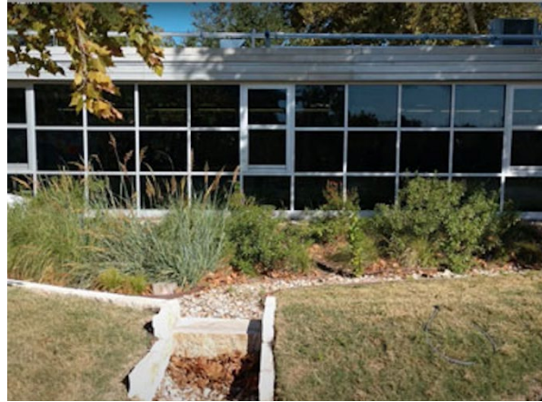
Reilly Elementary: Rain-catching landscape
