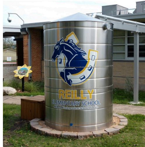
Reilly Elementary: Cistern to capture stormwater
